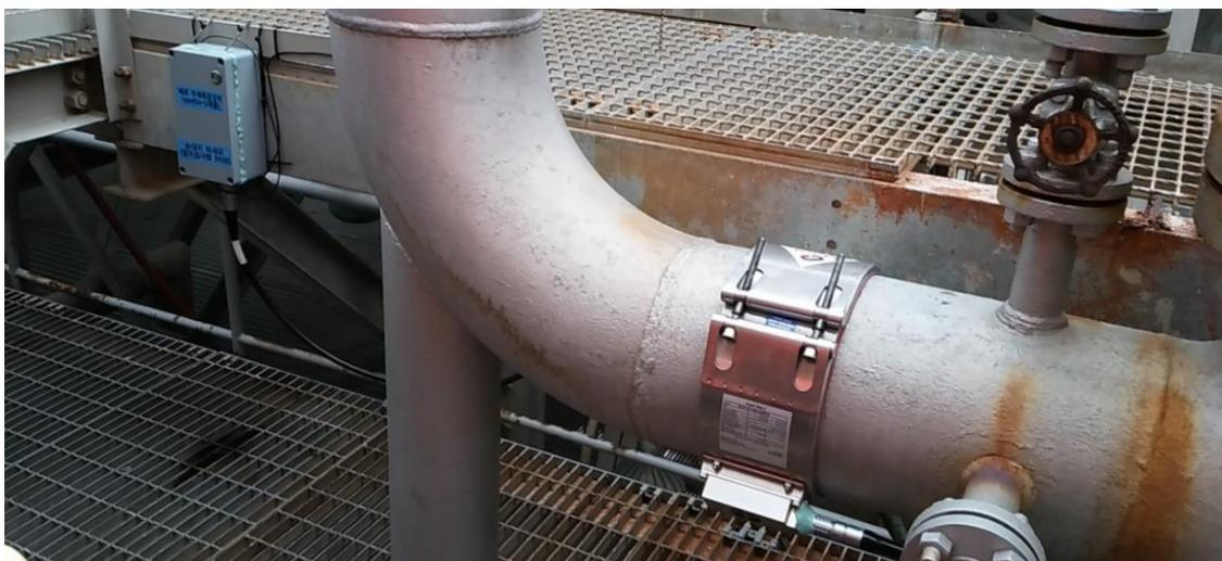
**Figure 4** Example of SpotOn<sup>®</sup> U installed at pipe in Aromatic unit
